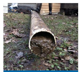
A neglected perimeter pipe causes mud build up and makes it difficult for water to pass through.
