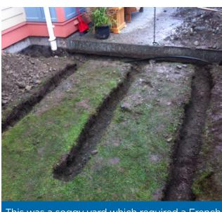
This was a soggy yard which required a French drain, this is the beginning of the installation process.
